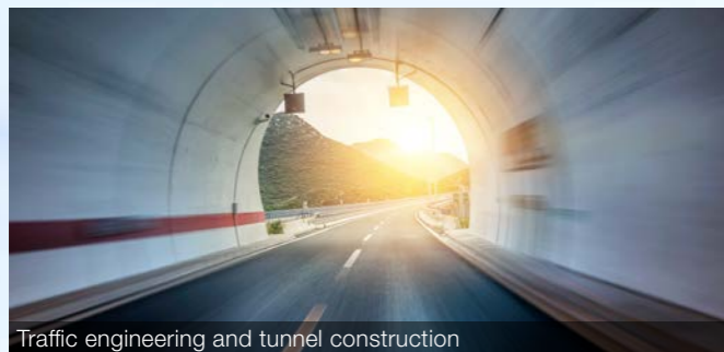
Traffic engineering and tunnel construction
